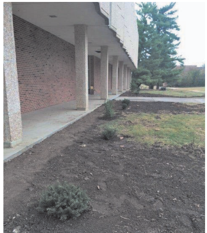
New shrubs installed in front of Thompson.
